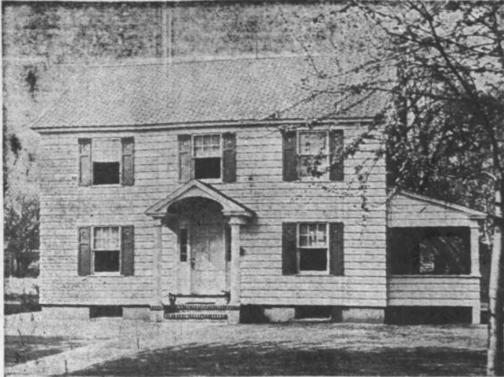
This New England Colonial is the new home of Dr. and Mrs. Charles F. Fasce. It is located on Andover Street and was built by Contractor James J. Quirico.
