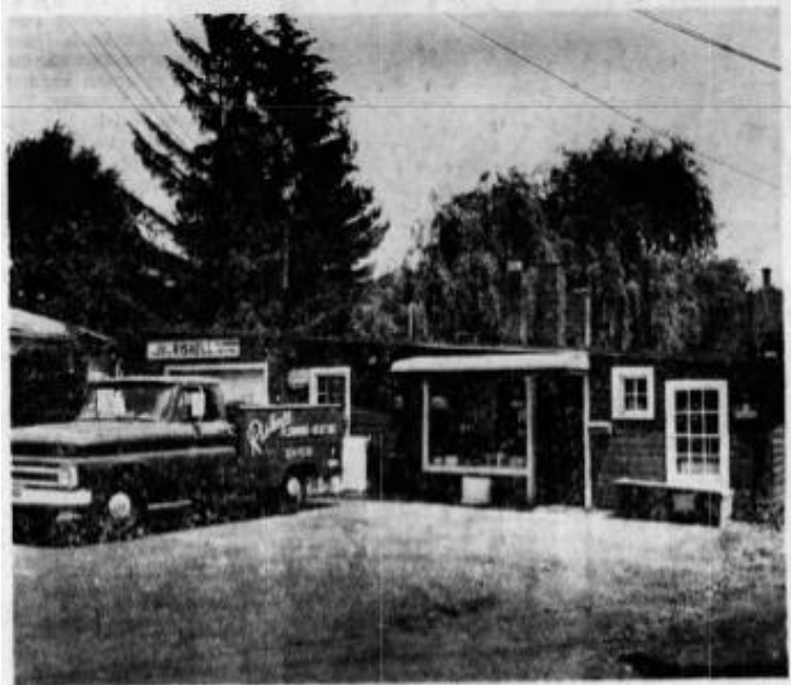
NAMCO APPROVED —Rishell Plumbing & Heating, Inc., located at 12 Brownson Street, Binghamton, has earned the Namco Seal of Approval through their strict adherence to the Namco Code of Ethics. Rishell Plumbing & Heating, Inc. specializes in all types of plumbing jobs, both big and small.
