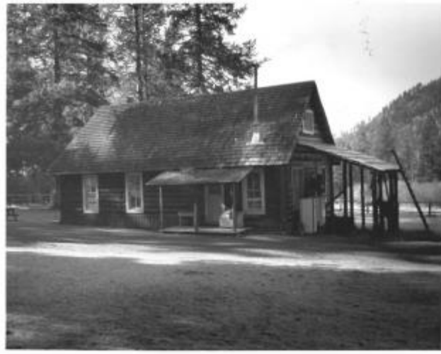
1) Moose Creek Ranger Station 2) Idaho 3) James Heid 4) October, 1989 5) Nez Perce N.F. Supervisor's Office 6) Building #1 facing west
