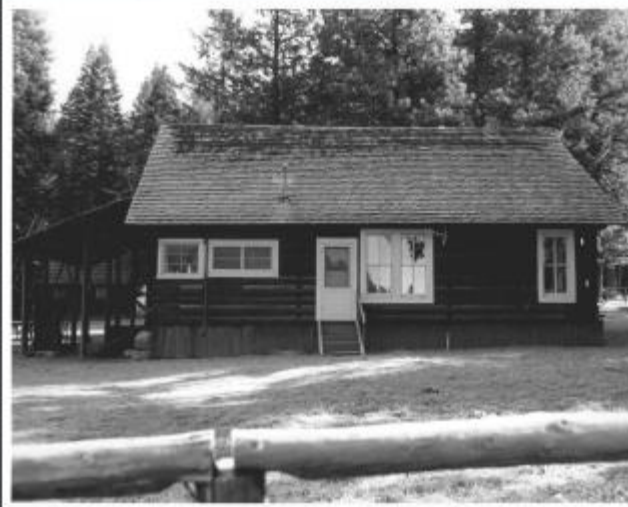
1) Moose Creek Ranger Station 2) Idaho 3) James Heid 4) October, 1989 5) Nez Perce N.F. Supervisor's Office 6) Building #1 facing east
