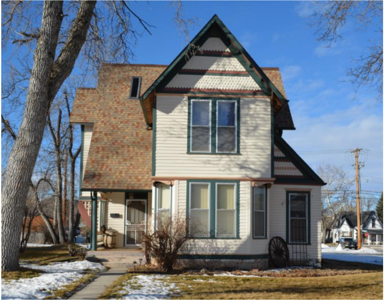
Built in 1887, the John and Elsie McMillan House is listed on the National Register for its local significance in Architecture. It is a good example of the Queen Anne Style and one of the few Victorian influenced homes in Sturgis that retains high integrity. Click on image to view larger.
