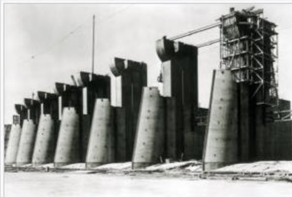
Fort Peck Dam spillway construction. Gate piers No. 3-9 completed. Pouring No. 10. Fort Peck, Montana
